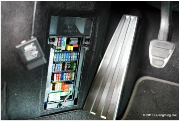
Above: View of the fuse box area (981, others similar)
