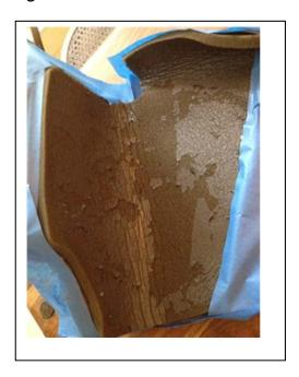
First, I taped if off with wide blue painter's tape (R) to avoid overspray on carpet. I wanted to loosen the flaking pieces off before I sprayed it. I tried a Teri-cloth towel- just flaked more up. Tried vacuum with small attachment- still *no joy*.
